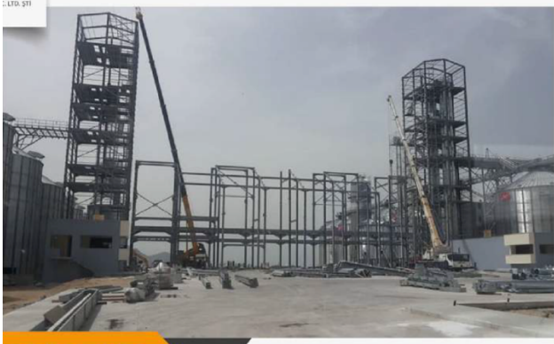
PanCihan steel structures under construction
